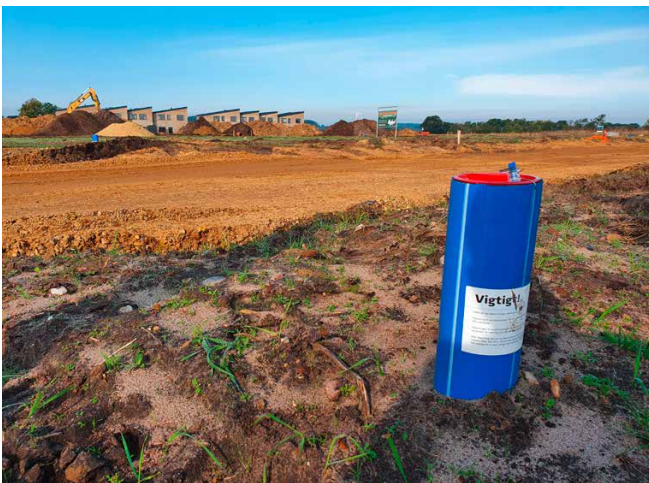
Temporary inlet on a new construction site with a sensor installed in the lid.
