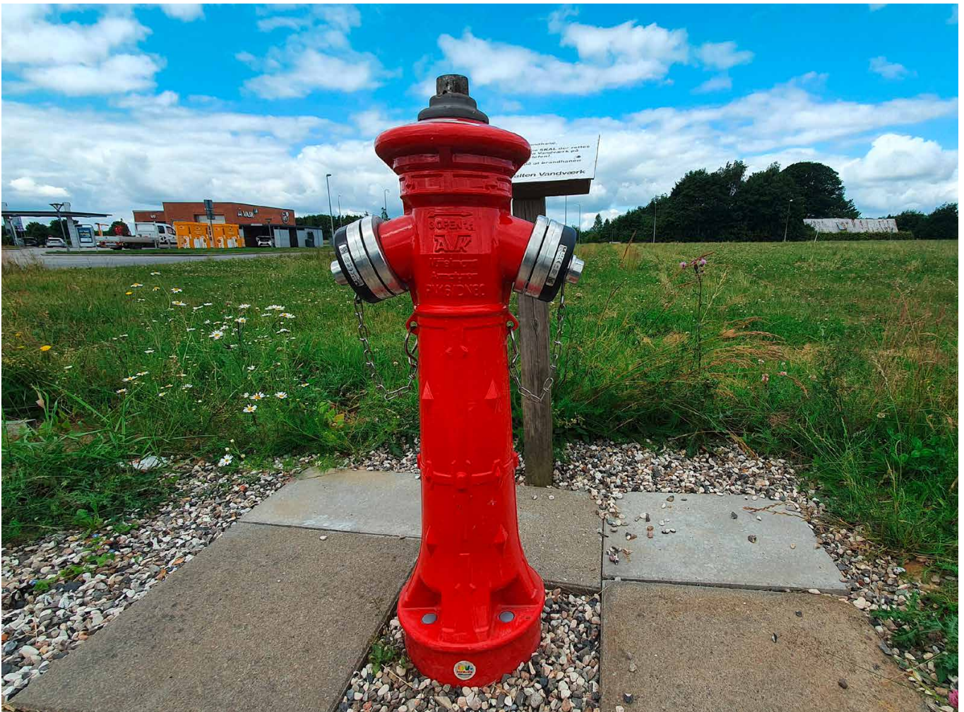
Hydrant with VIDI Caps installed. The use of a hydrant deeply affects the pressure in an area. Therefore, it is important for the utility to know when the hydrant is being used in order to distinguish between a pressure drop coming from regular use or from a pipe burst.
